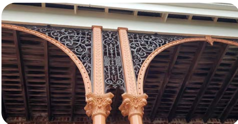
New balustrade installed at Cooktown Museum
