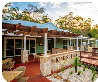
The Homestead Opened June 2024
