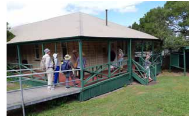
Festival visit to Stradbroke Island and inspecting the remaining Building Ward 13 of the NSI Asylum, heritage listed in 2021
